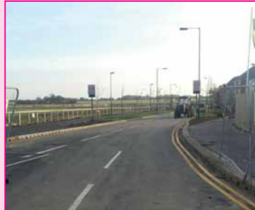
The completed Kingswood Parks side
