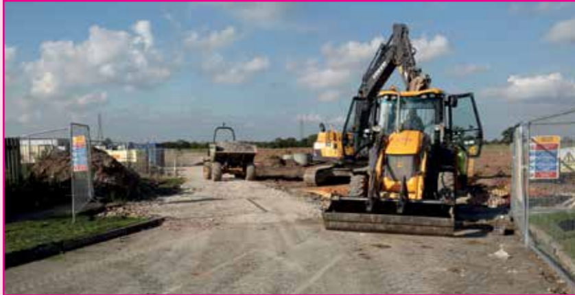
Construction on the Kesteven Way side of the link road
